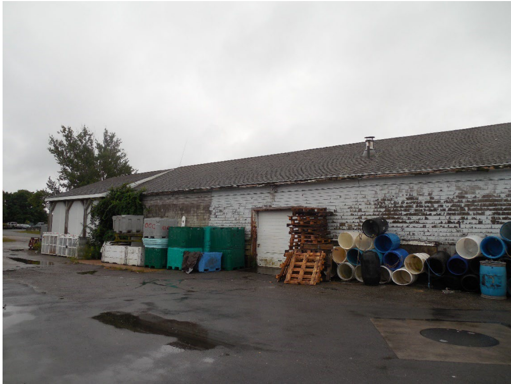
Operations Building – North Elevation (Photo #5)
