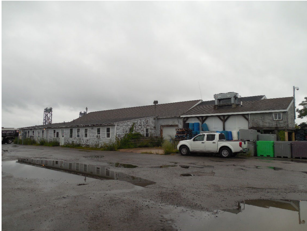
Operations Building – South Elevation (Photo #9)
