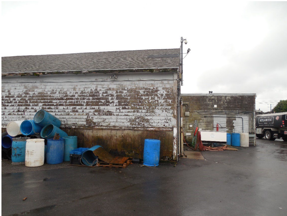
Operations Building – North Elevation (Photo #6)
