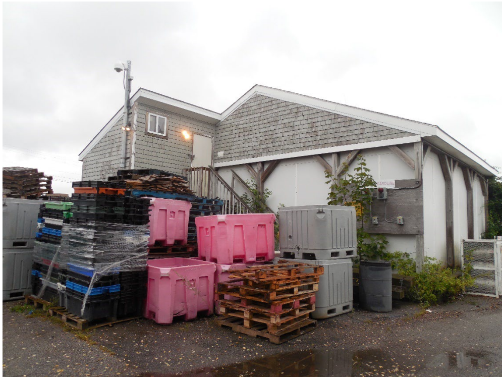
Operations Building – East Elevation (Photo #4)
